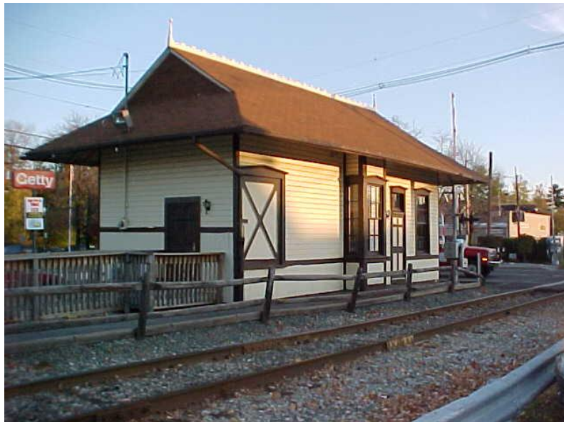
View of original railroad station for the NYS&W at Diamond Bridge Road.
